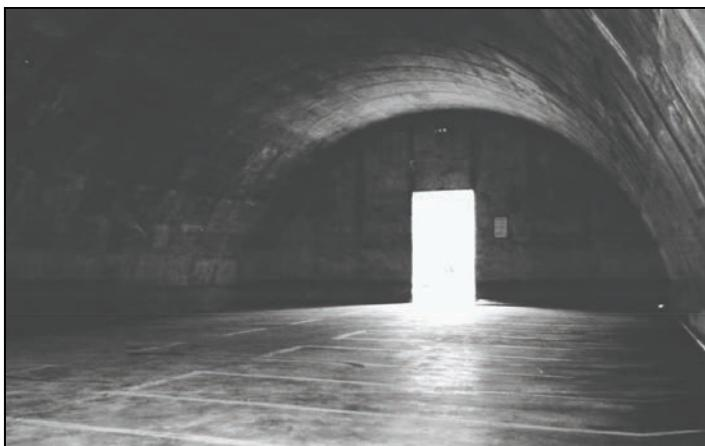
Igloos at KSAAP were built for storage of components and finished products, prior to being shipped. Pictured above is the interior of the units, which were constructed of reinforced concrete and covered with two feet of earth. There are 95 igloos at KSAAP, each measuring either 1220 sq. ft or 1813 sq. ft. They
